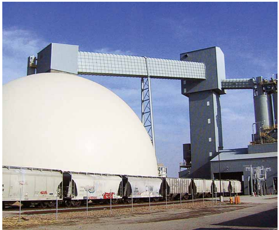
California Portland Cement Co. - Stockton, California
